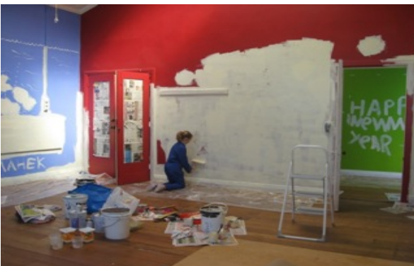
From this to this
