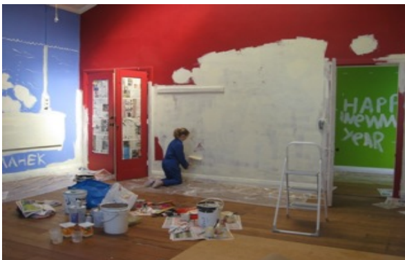
From this to this
