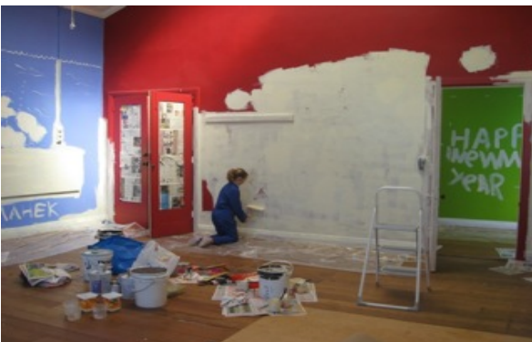
From this to this
